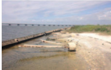
Unless the causeway's toppling sea walls are reinforced, this nesting island will return to the bay.
