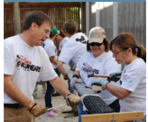
Bottom: Disney VoluntEARS helping with improvements maintenance of a flight barn.
