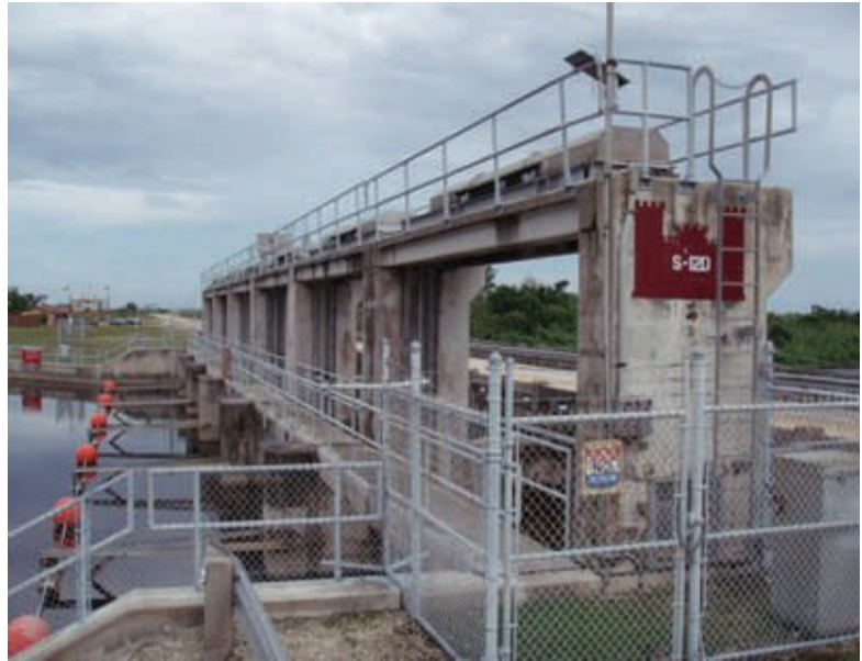
The S-12D structure along Tamiami Trail controls flows into Everglades National Park Photo by Robert V. Sobczak, Big Cypress Nat'l Preserve Hydrologist
