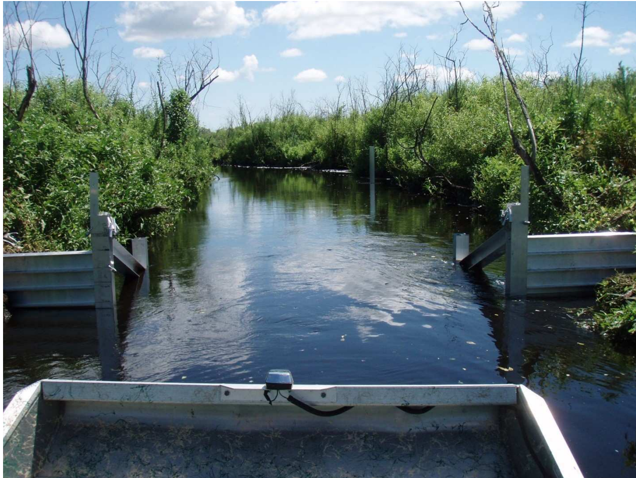
Flowblock from West (photo taken on 8/20/10)
